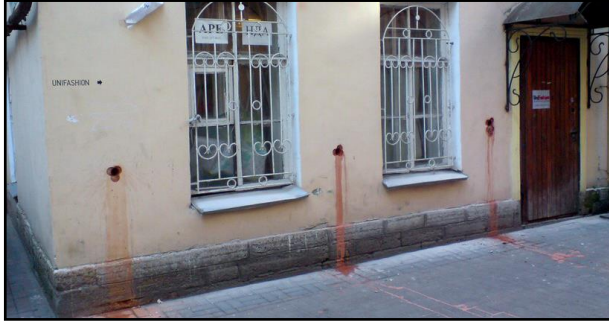
Figure 4. Sampling sites from building walls to the address: Nevsky prospect 136
