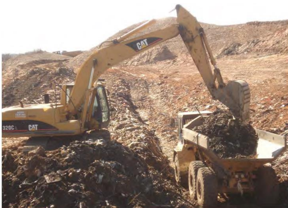
Figure 8: Waste excavation (FDEP, 2009 [17])
