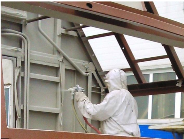
Figure 1. Locomotive - 2ТЭ25КМ. Application of the coating on the internal surface of the cabin
