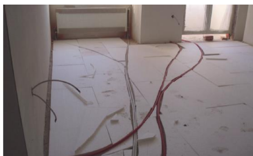
Figure 4. (a) Typical error in workmanship - broken insulation, (b) Possible solution when there are too many cables and pipes (1-reinforced concrete slab, 2-rods, 3-slab, 4-flooring)
