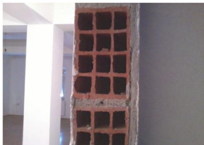
Figure 6. Typical errors in workmanship; (a) irregular mortar layers, (b) vertical joints not filled with mortar
