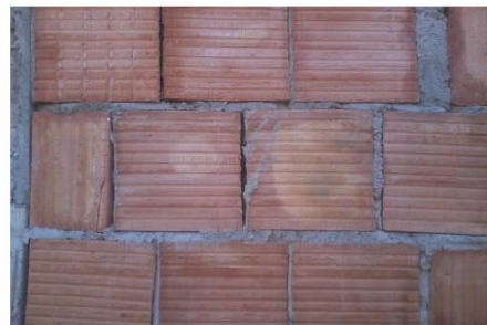
Figure 6. Typical errors in workmanship; (a) irregular mortar layers, (b) vertical joints not filled with mortar
