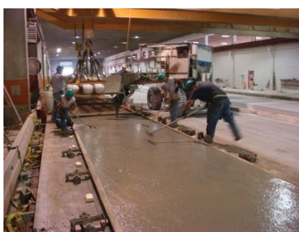
Figure 37. LaBahn Arena, Wisconsin, USA - Concrete pour into precast bed complete [71]
