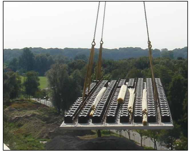
Figure 2. Example of Airdeck slab construction [2]
