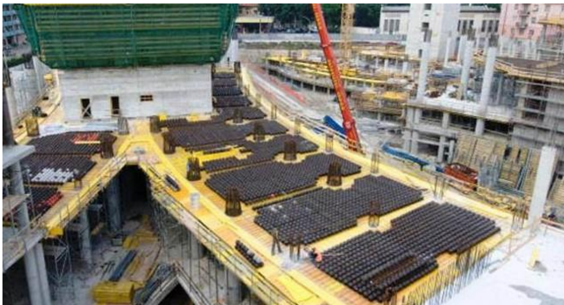
Figure 21. Altra Sede, Milan, Italy. Cobiax technology [66].
