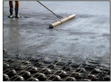
Figure 12. Concreting slab on site [5]
