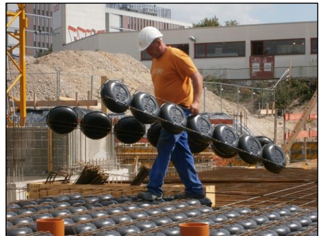
Figure 4. Example of installation of Cobiax slab [7]
