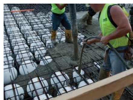
Figure 38. LaBahn Arena, Wisconsin, USA – Construction workers pouring concrete over the bubbles to form the reinforced slab of steel, air, and concrete [71]
