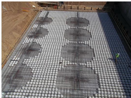
Figures 34, 35. LaBahn Arena, Wisconsin, USA. BubbleDeck [70]
