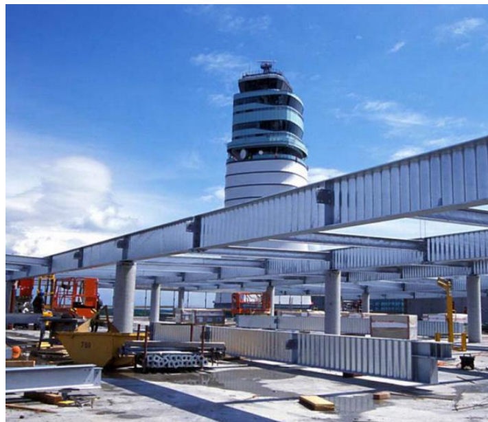
Figure 6. Parking ramp at the airport in Vienna, Austria. As joists used steel beams with wavy-wall corrugated production company Zeman. [6]
