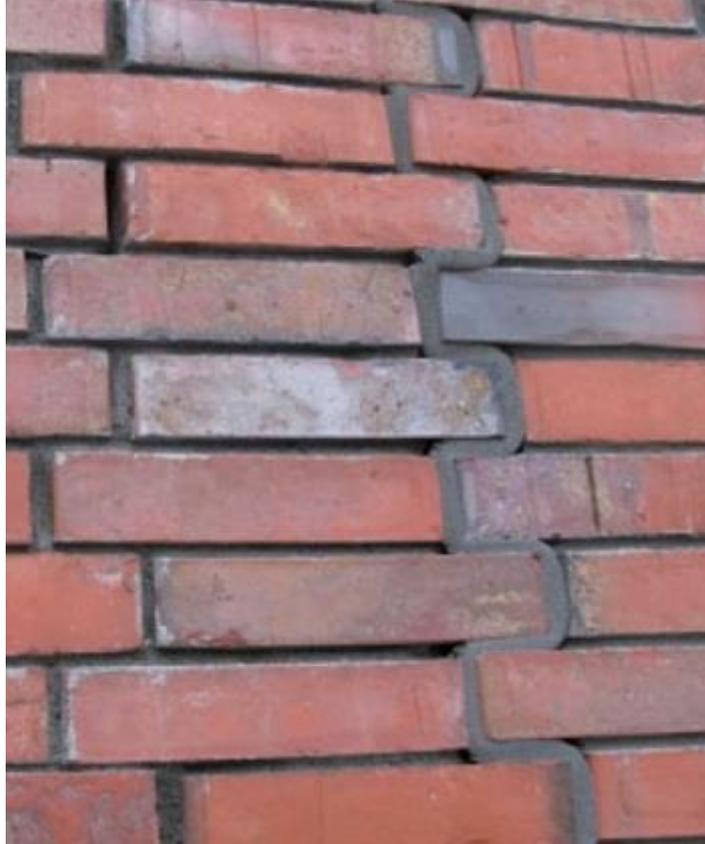
Figure 1. Example of tothing joint construction
