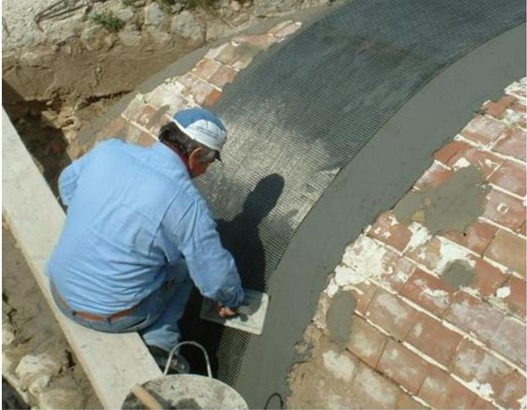
**Figure 3. Carbon fiber net placement on reinforced masonry vault**
