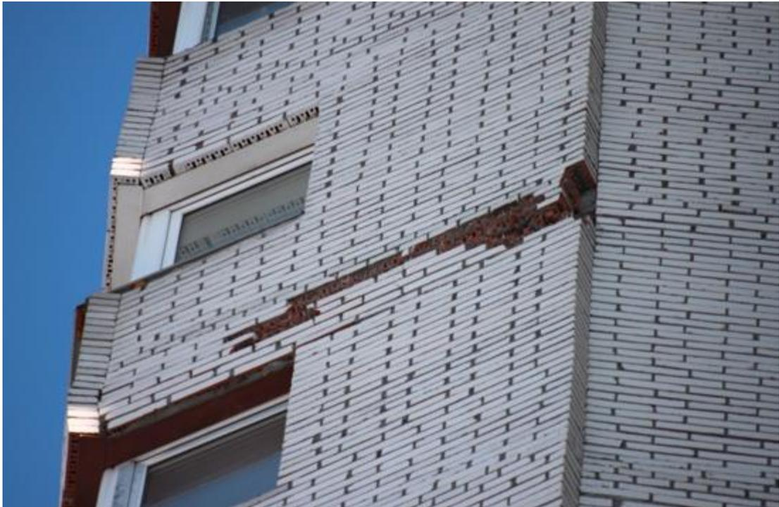
Figure 2. Degradation of surface layer made from high voidage with low frost-resistance
