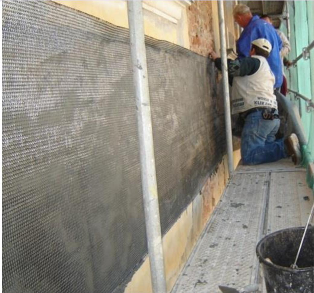
**Figure 4. Strengthening brick wall by reinforced plaster**
