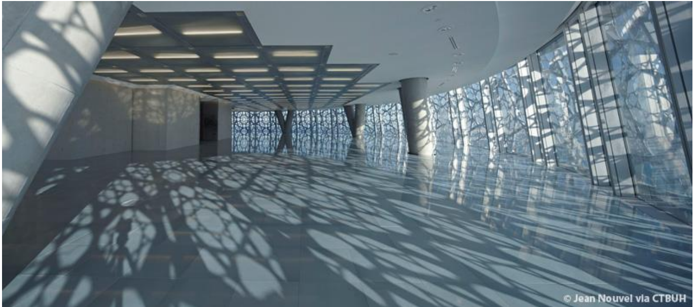
Figure 3. One of the premises in Doha Tower. Frame is made of crossed metal parts, which are superimposed on each other and prevent the rooms from overheating [18]
