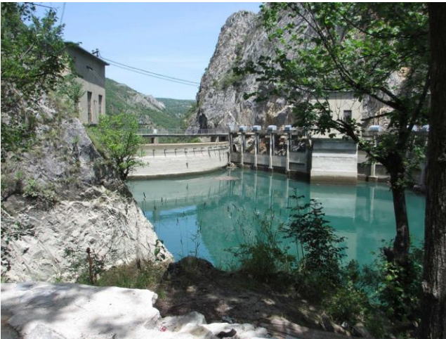
Figure1. The arch dam Matka on a river Treska
