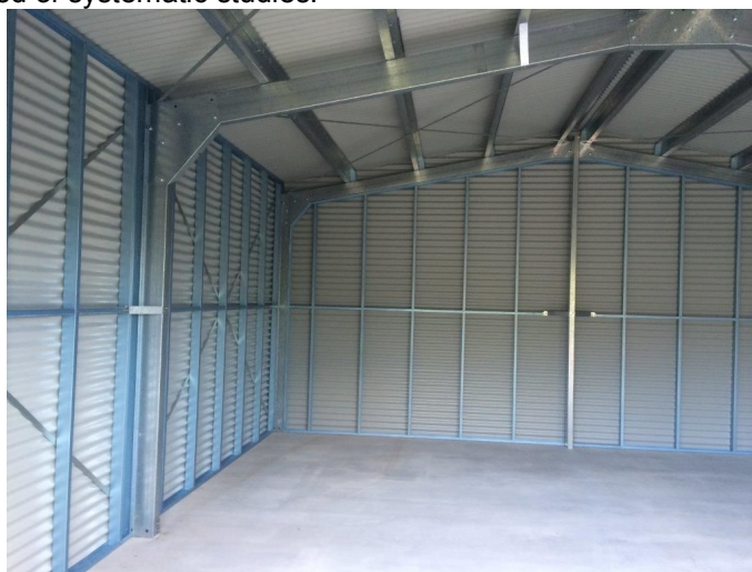
Figure 3. CFS profiles working as flexural elements (girders and purlins)
