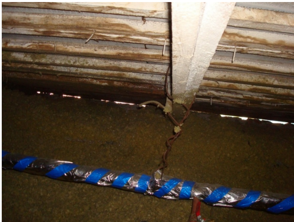
Picture 2. Inlet air holes at the cornice
