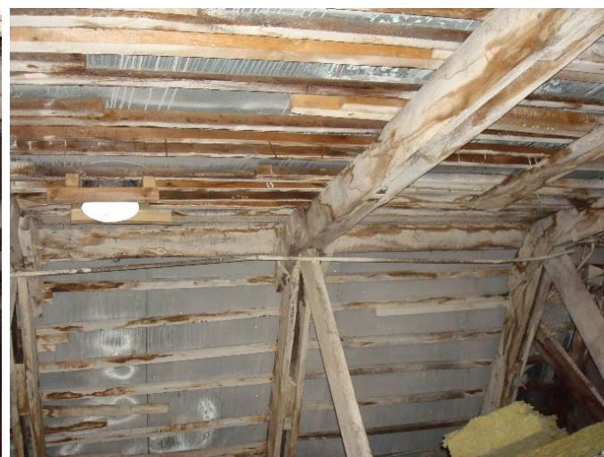
Picture 5. The cowls in the roof structure
