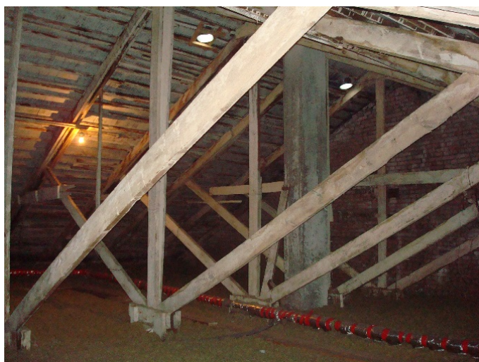
Picture 4. The cowls in the roof structure
