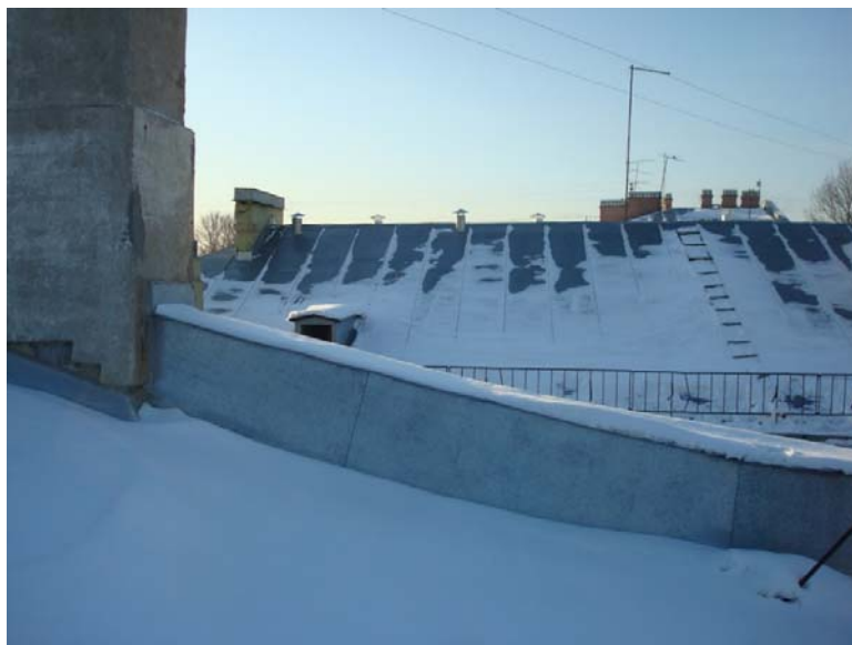
Picture 6. Exhaust holes (view from the roof)
