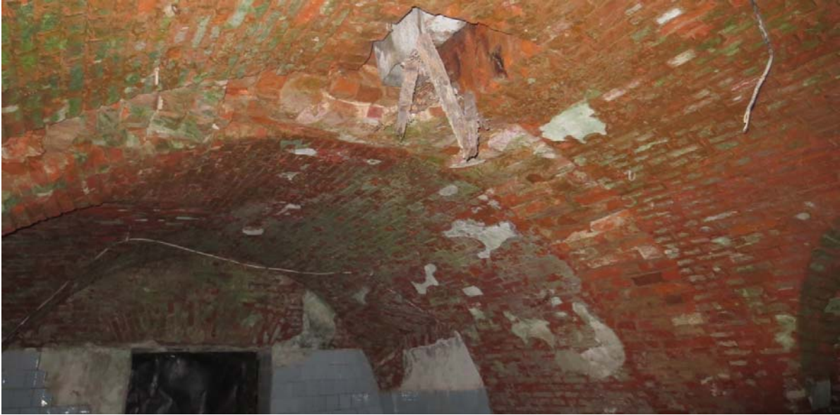
Figure 2. Dividing arch with a different structure of masonry
