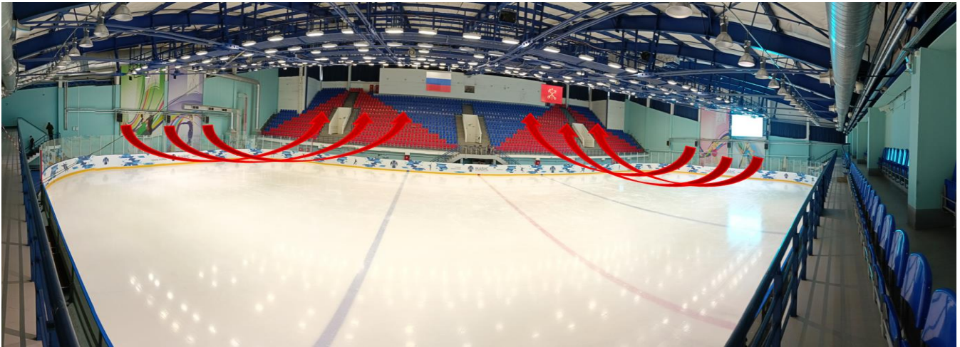
Fig. 3 – Scheme of distribution of air flows of fan heaters over the ice arena (photo taken by the author)
