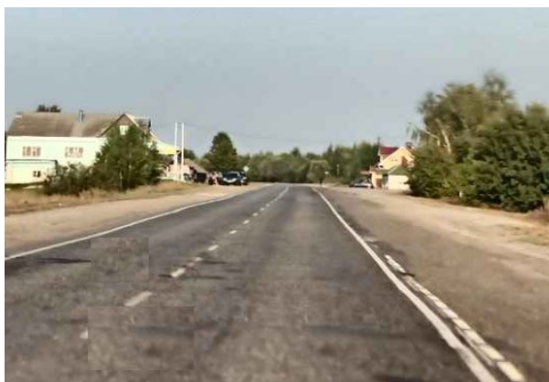
Fig. 1. - Section of the road R-177 « Povetluzhe » in the village of Arda
