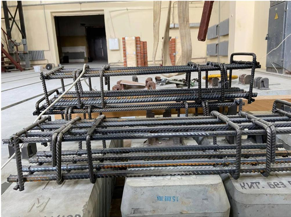
**Fig. 2 - Reinforcement of the half-step**
